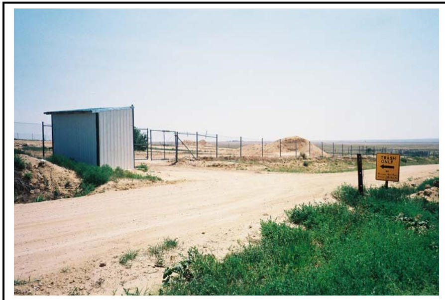
View looking southeast of the Haswell landfill.
